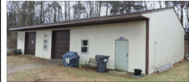
LARGE BARN HEATED SHOP
